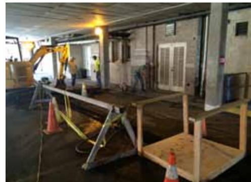
Plumbing work under covered parking area
