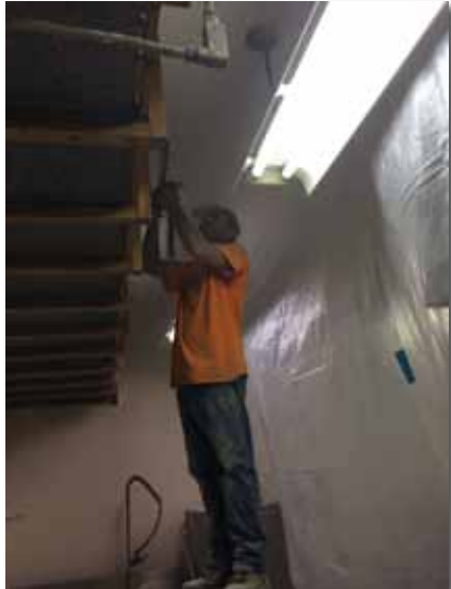
HVAC work in the kitchen
